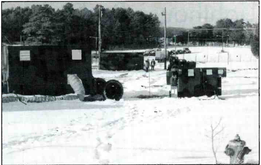
Here are the truck-mounted modules for the Army's portable AM station. Left: the transmitter unit with self-contained HVAC and generator. Center (rear-most, next to pole): a camouflaged studio building. Right (next to transmitter unit): a generator.
