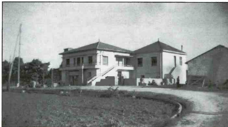
The AFHQ "Hippo" 50-kW mediumwave transmitter was on the ground floor of the center farm building near Port d'Esu, Algiers. (Courtesy John R. Hall, W5ETK.)
